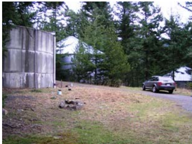
Rosario Utilities Water Storage Reservoirs
