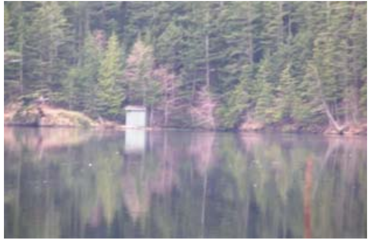
Rosario Utilities Water Intake on Cascade Lake
