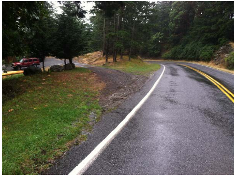
Figure 22. Photo of Stormwater Flowing from Rosario Road into a Private Drive.
