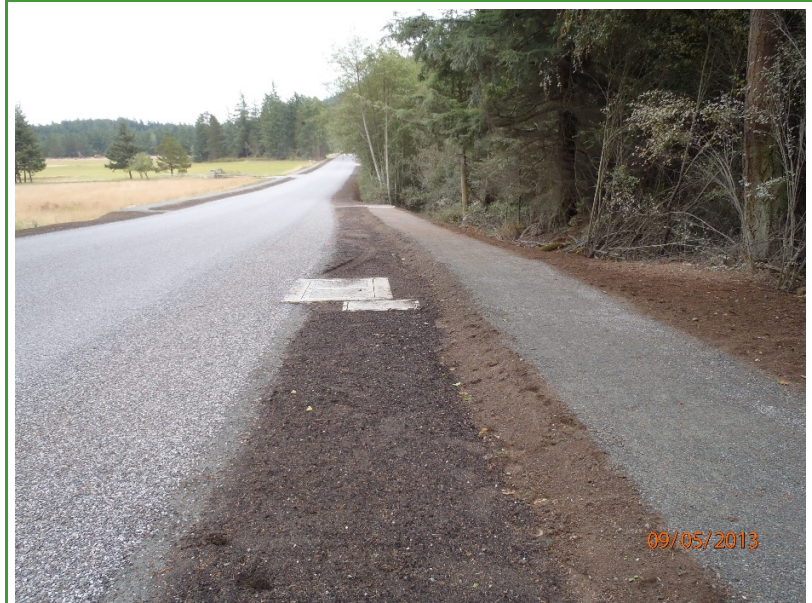
Figure 23. Narrow Area Vegetated Filter Strips for Filtration and Treatment Were Used to Improve Stormwater Quality Coming From Mount Baker Road, Orcas Island.
