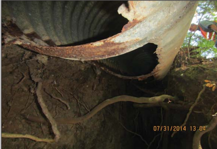
Eroded pipe at Olga Road
