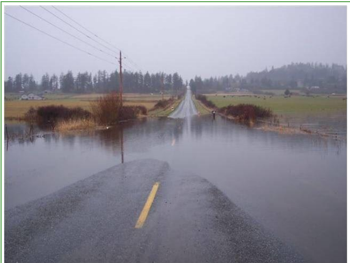
Figure 1. Flooding Over Bailer Hill Road.
