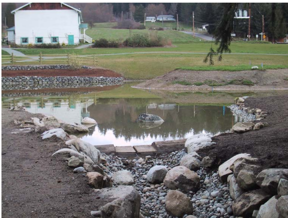
Figure 19. Sawn Log Weir with Horizontal and Vertical Notches.
