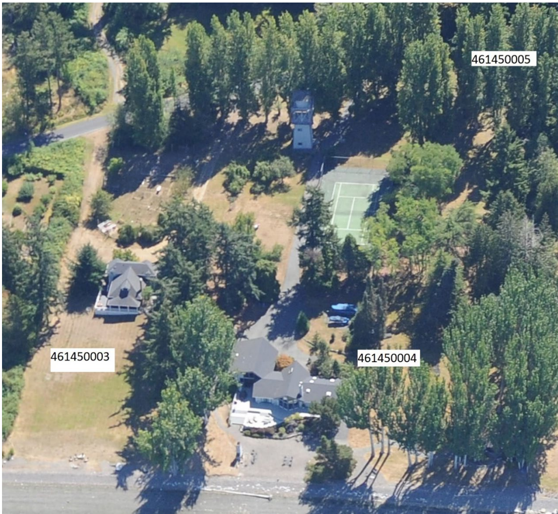
The primary structures pictured above have been demolished.
