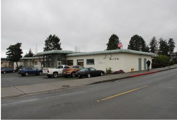
Figure 10. The east (left) and north (right) elevations of the Courthouse Annex building.
