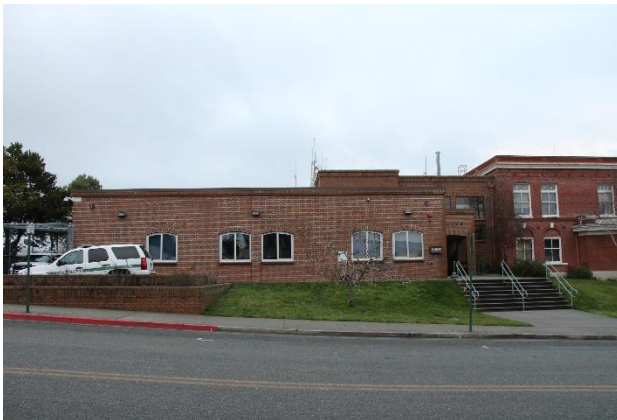
Figure 6. West elevation of the 1996 one-story Sheriff Wing addition.
