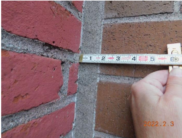
Figure 21. Mortar-filled gap between the original courthouse building and the 1980s expansion.
