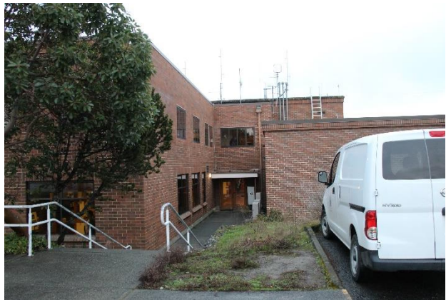
Figure 7. Looking south towards the two-story Courthouse expansion (left) and Sheriff Wing addition (right).
