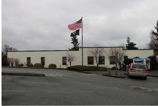
Figure 11. The west elevation of the Courthouse Annex building.
