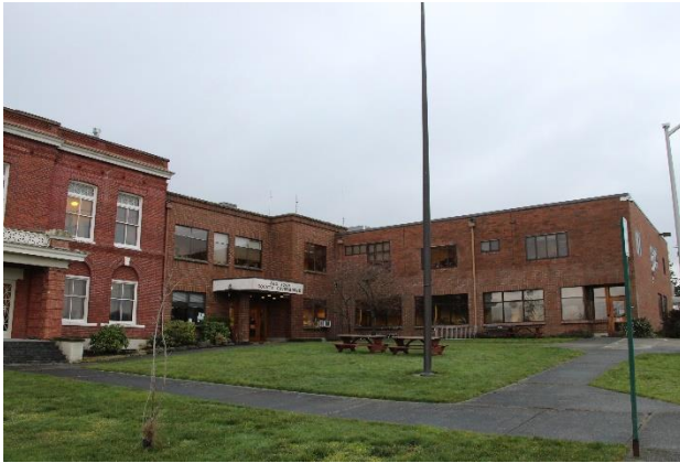
Figure 4. South and east elevations of the 1980s two-story addition. The original 1906 Courthouse building can be seen on the south (left) side of the building.
