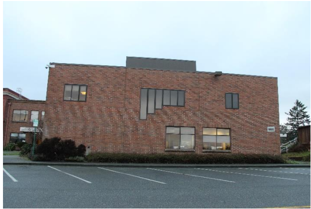
Figure 5. East elevation of the 1980s two-story Courthouse expansion.
