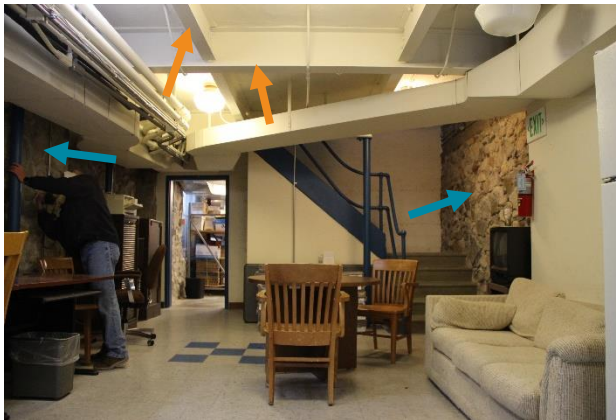
Figure 19. View of the Courthouse basement. Note the steel beams (orange arrows) supporting the floor above and stone walls (blue arrows) on the east and west sides of the basement.
