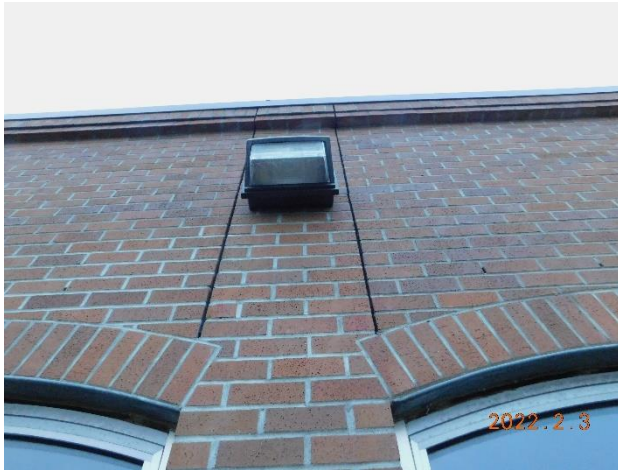
Figure 26. Sheriff's Wing, expansion joints and weep holes in masonry veneer.
