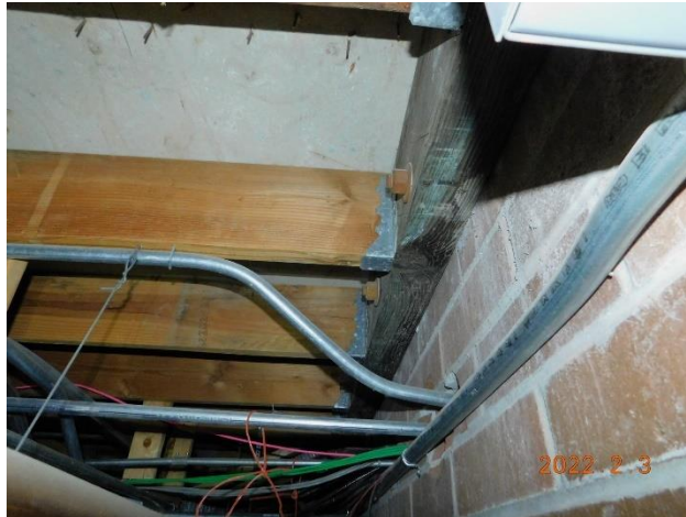
Figure 23. Typical floor framing-to-wall connection.
