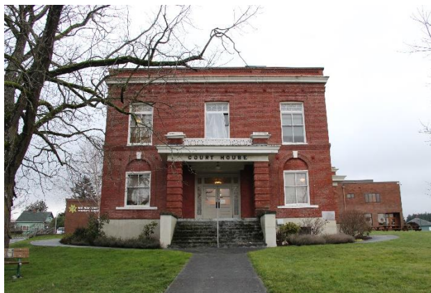
Figure 2. South elevation of the original 1906 Courthouse.
