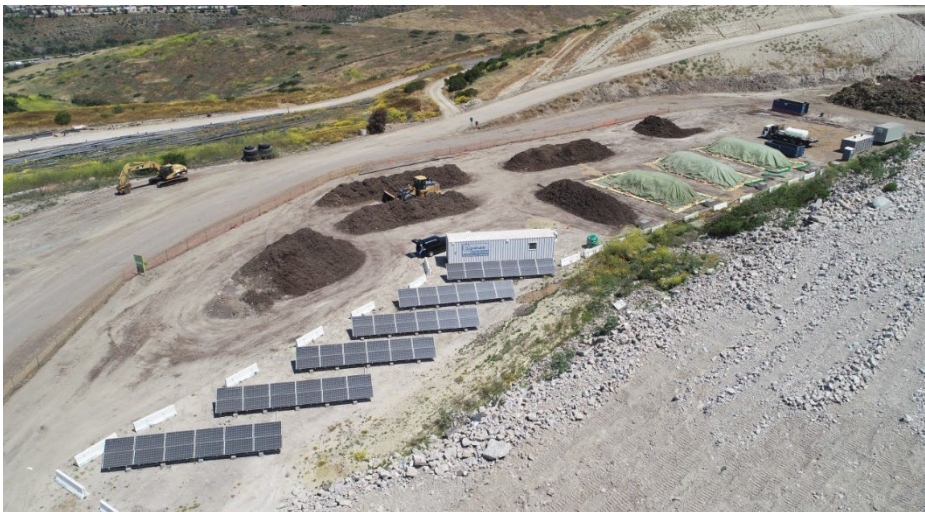
Demo Project using SG Mobile® System with GORE® Cover
