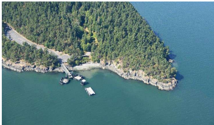
Lopez Island Ferry Terminal
