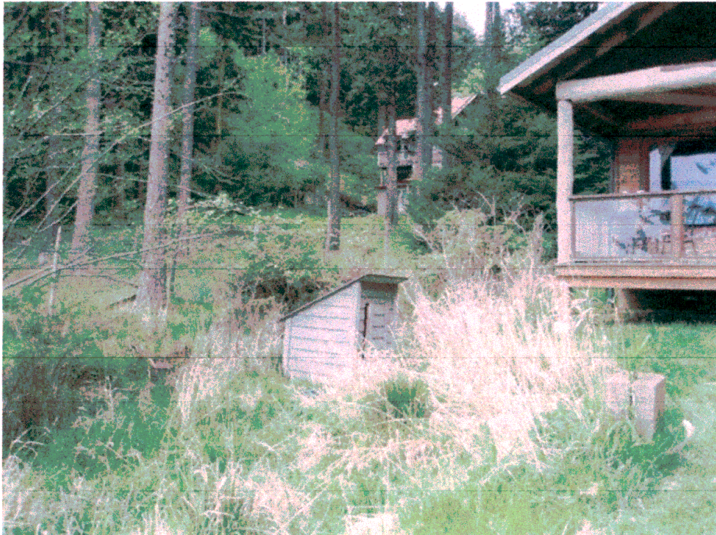
Corner of Cabin Spring Pumphouse Yard Fence Main Residence
