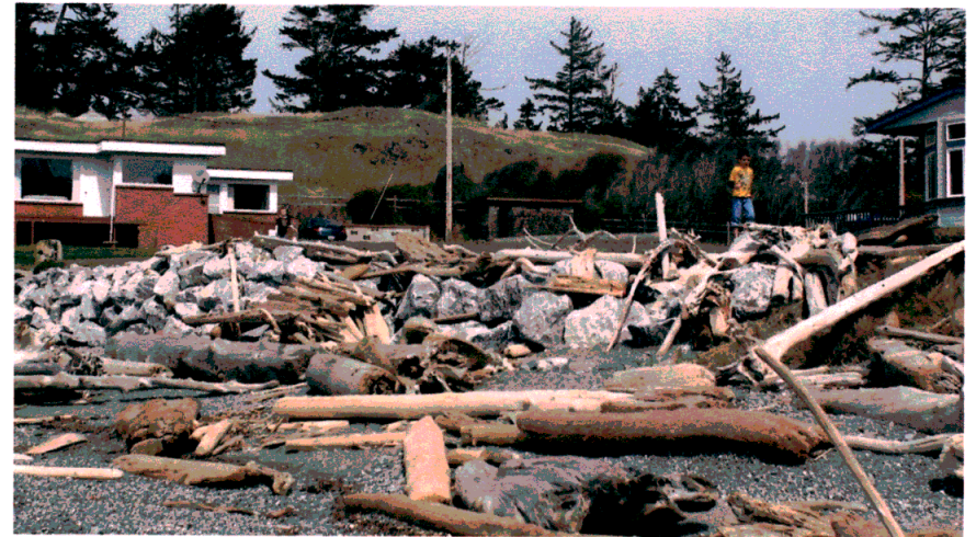
Breakwater for 1608 & 1631 Mackaye Harbor Road
