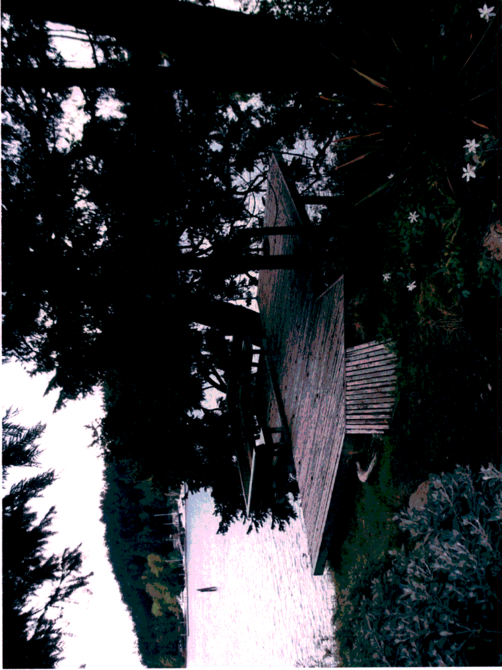
View of existing sun deck on extreme SE corner of lot, footings land on Existing concrete bulkhead below
