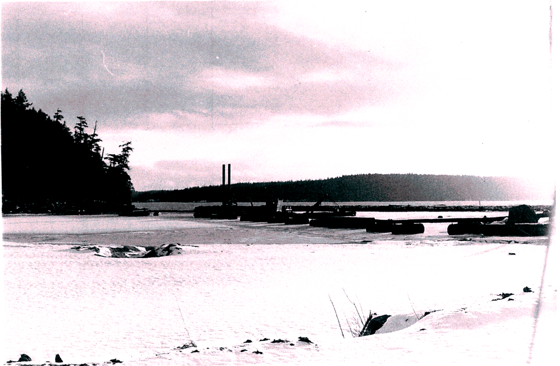
Winter 1968 -1969 Ice on the water, cutterhead dredge with two discharges.
