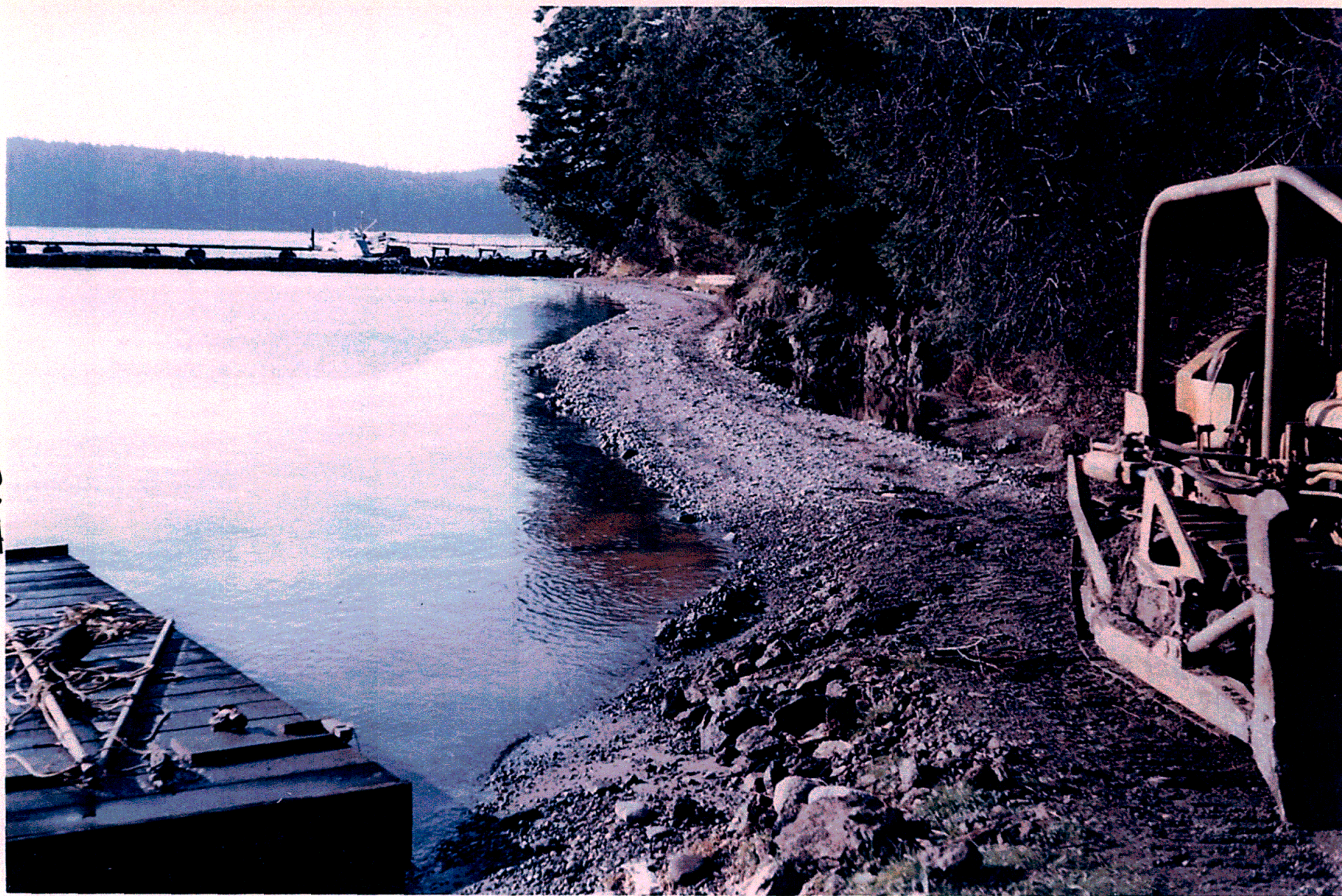
Haul road to dump rock for break water. note outfall on bay side of beach
