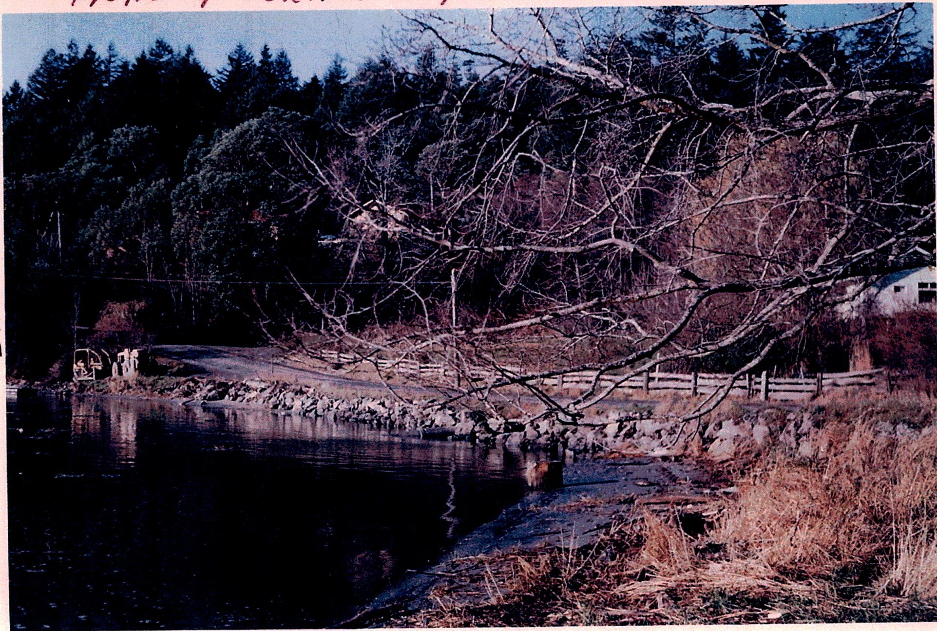
Exton Equipment - 1968 - building road for breakwater. Note pond outfall.
