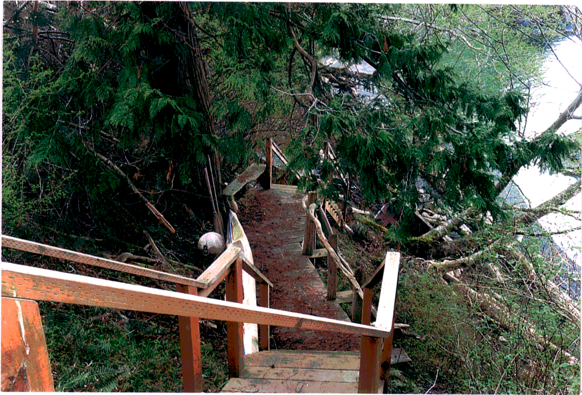
This picture shows the stairs leading from the Gutschmidt main house to the pocket beach on parcel # 272334004 being actively used by the Gutschmidt family.
