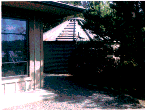
Catchment Water Tank behind Garage
