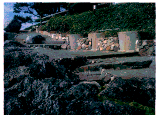
TANKS WITH CONCRETE VAULT BELOW
