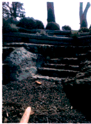
Stairs on West Gully
