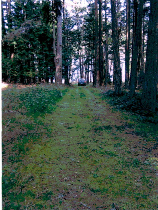
PHOTO 10 (4-22-12) – GRASS COVERED GRAVEL ROAD - Looking down at truck parked above ramp. Road located on road easement.
