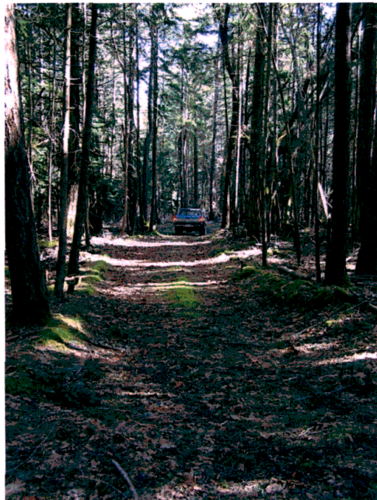
PHOTO 12 (4-22-12) – GRAVEL ROAD - Located on easement. This section of road was built over an existing logging road.
