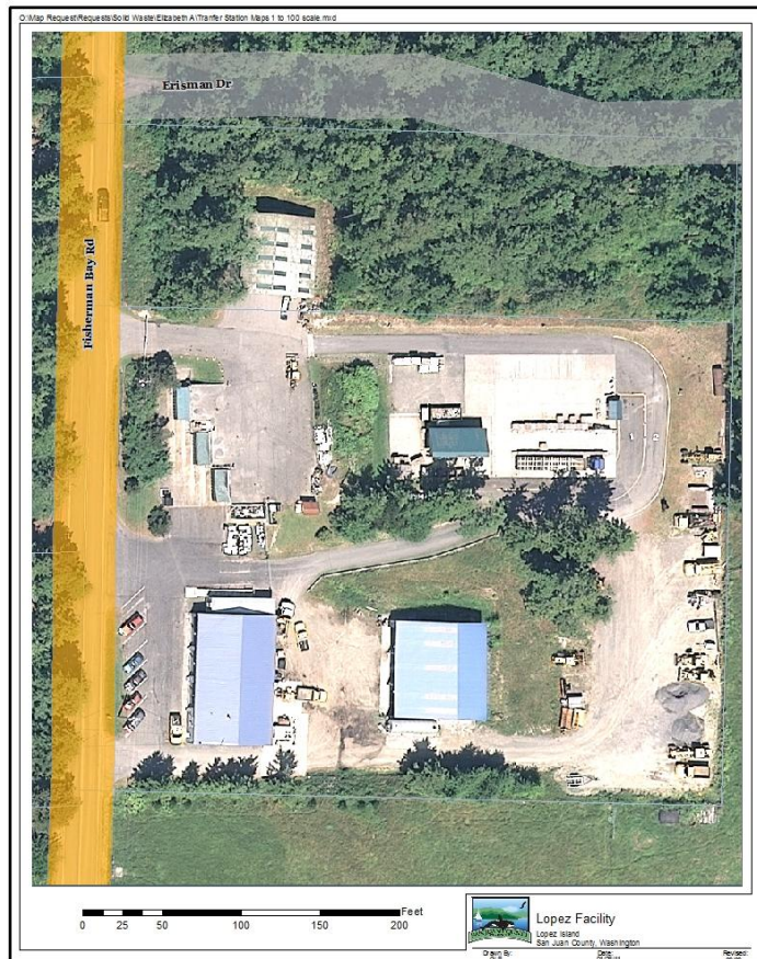
Figure 6.3 Lopez drop box facility
